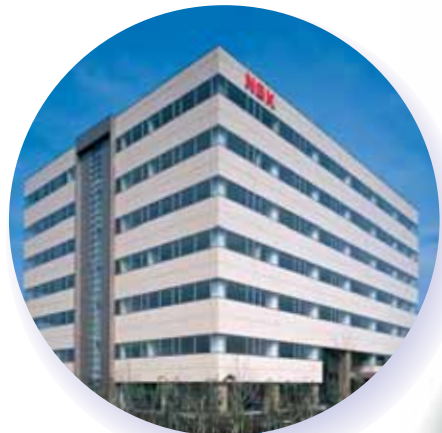
Bearing Technology Center (Japan)
