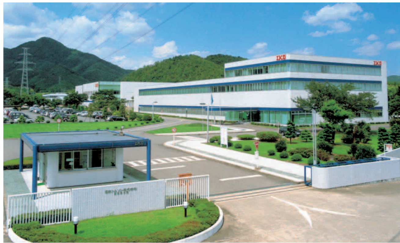
Main entrance of Gifu plant
